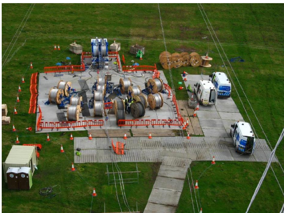
Plate 4.3 conductor pulling position and drums
